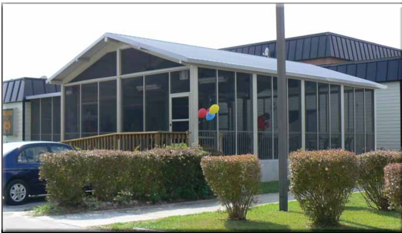
Illini, with wall system
